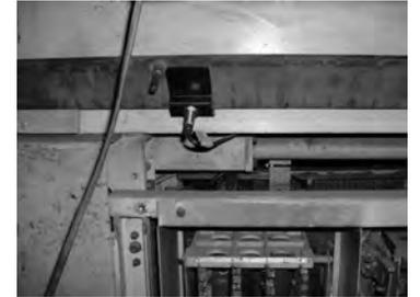
NOTE: The electrical purpose of each sensor is supplied in case the sensor is replaced with a different type of a switch. When the sensor is not supplying ground it presents an open circuit. With the cable pointing up and the tab facing you, pin 1 is to the left. The wiring at pin 1 is 12VDC and pin 2 is ground. Pins 3 to 6 are the signal lines from each sensor as defined in the installation instructions.
